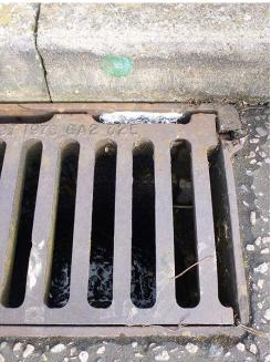
If required the Enkamat can be fairly easily removed from the gullypot at the end of the season by pulling away from the adhesive or cutting the Enkamat.
