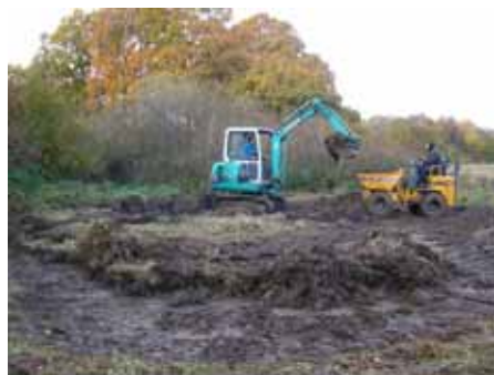
The start of pond creation work at Merrymeades, Photo by EARG
